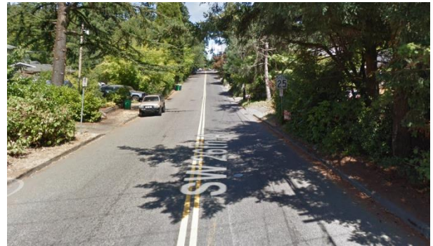
SW 26 th Avenue: I-5 Underpass to Taylors Ferry Road
